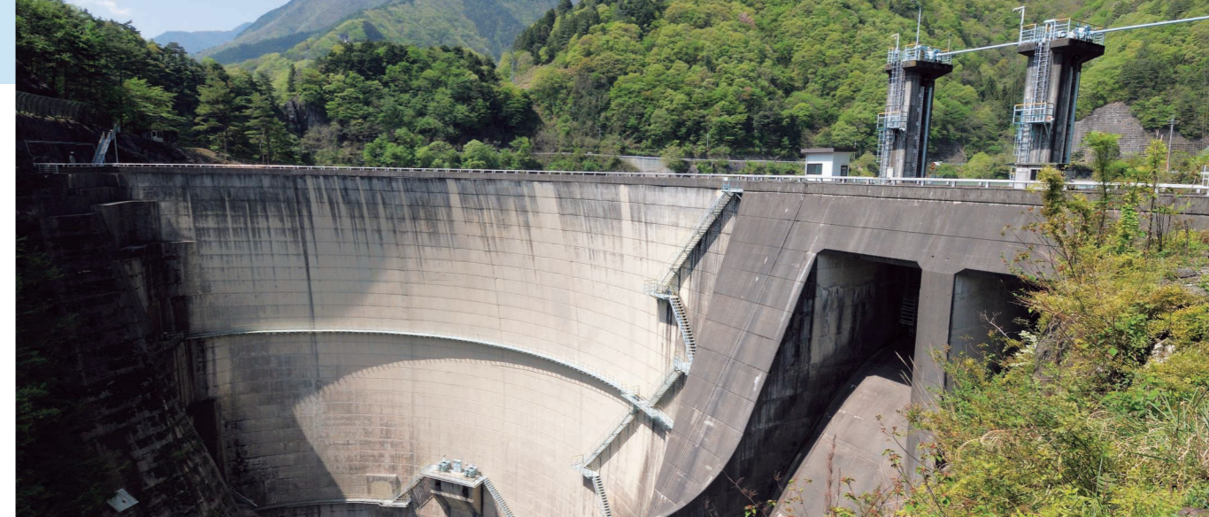
Amehata Dam (in 2009)
