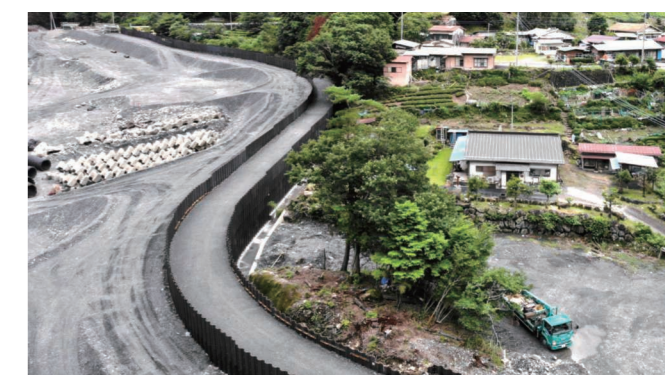
Temporary embankment under construction (in July 2020)
