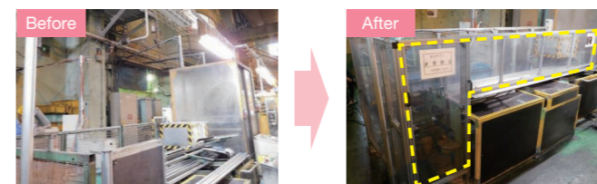
An improvement made at the Kambara Heat-Exchanger Plant of Nippon Light Metal Co., Ltd. The fence around the cutting machine was added, and an automatic cutout was installed.
