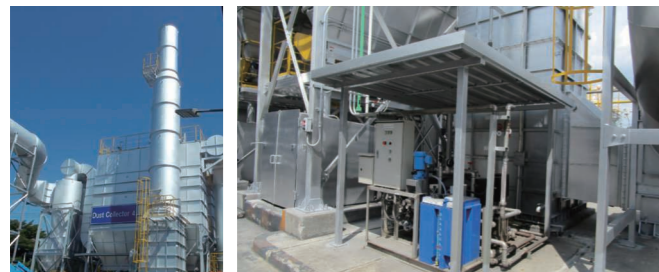
The Dust collector (left) and deodorizing equipment (right) of Nikkei MC Aluminum (Thailand) Co., Ltd.
