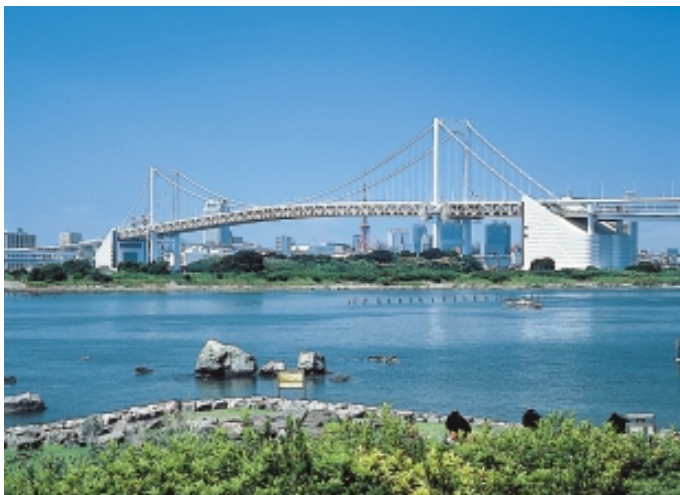
NLM’s Landscape Engineering Division manufactured the railings for Rainbow Bridge in Tokyo.
