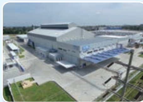
New Thai factory began operation in March 2017 (Chonburi Prefecture)
